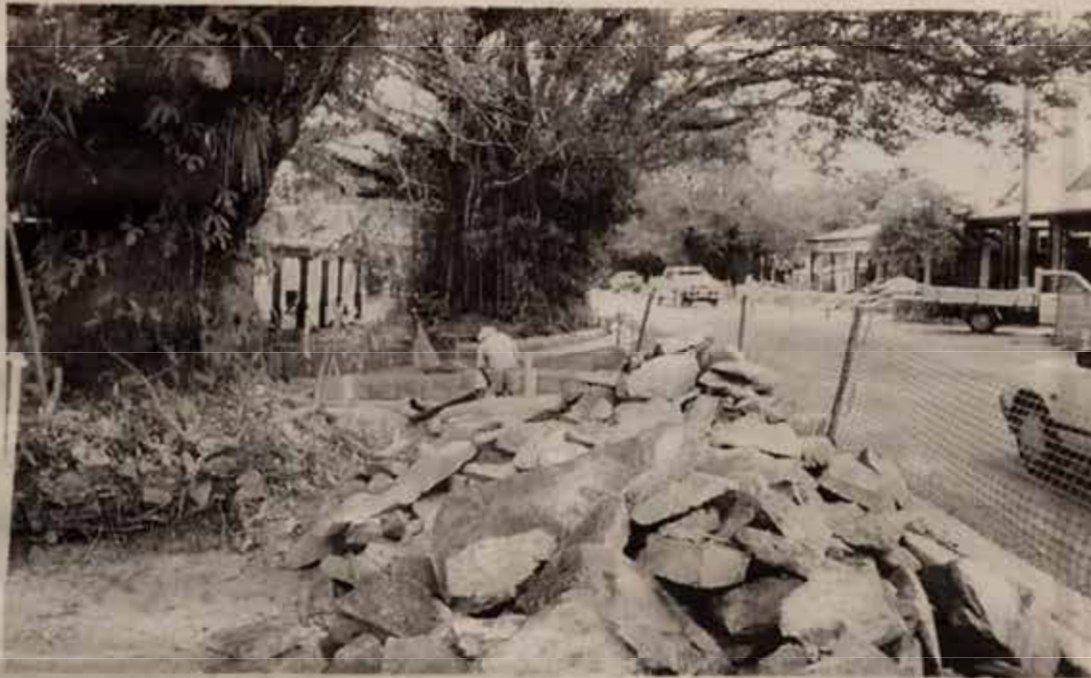
Ongoing works in Coondoo Street
