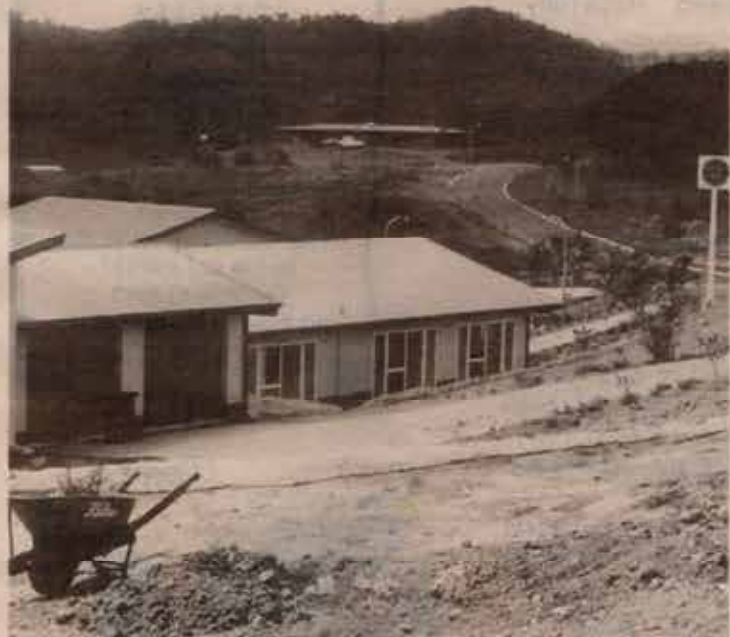
New Kuranda Ambulance Station, Fallon Road
