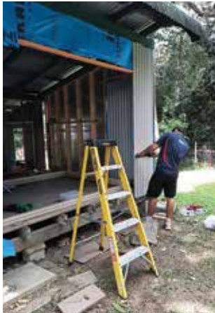
Work on the caretaker's cottage
