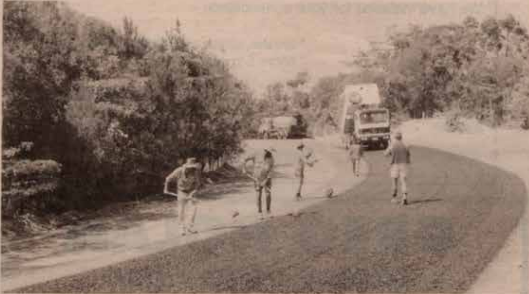
2km of sealing now completed making for a safer drive
