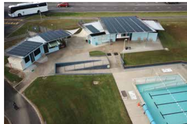
Solar installations at Kuranda Pool Barron River
