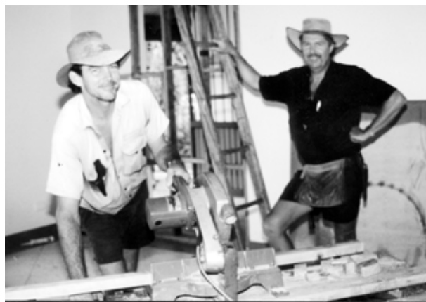
Phil Thorpe and Barry Isgar working at the new Visitors Centre
